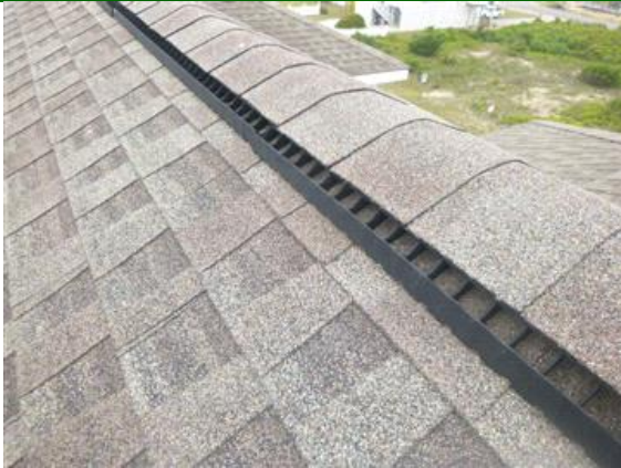
Exterior Of Ridge Vent
