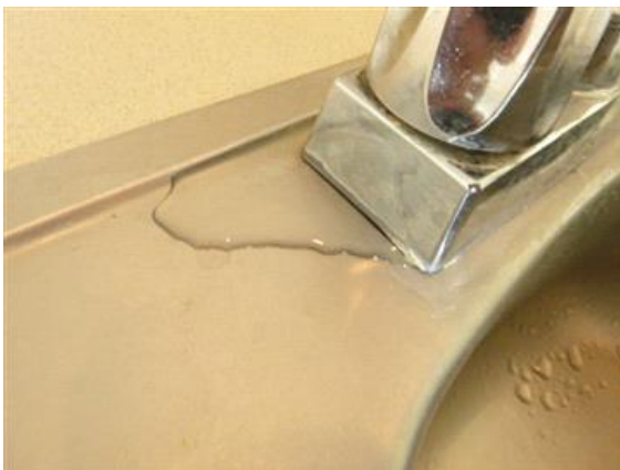
Leak At Bar Sink Fixture
