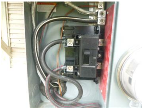
Main Disconnect Panel
