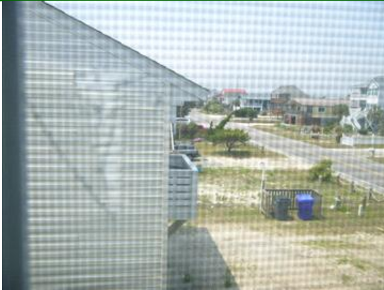
Damaged Window Screen
