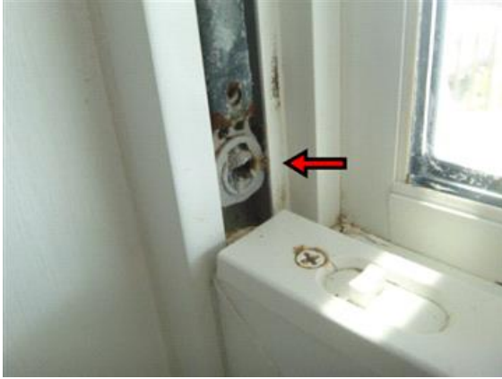
Sash Cord Mechanism Stuck
