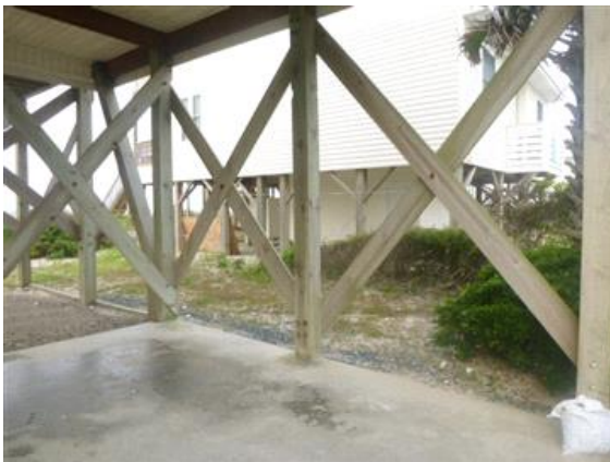
Typical Pilings With Cross Bracing
