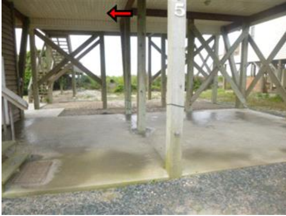
Obscured Floor Framing
