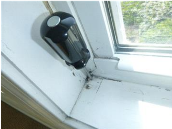
Decayed Window Sill Wood
