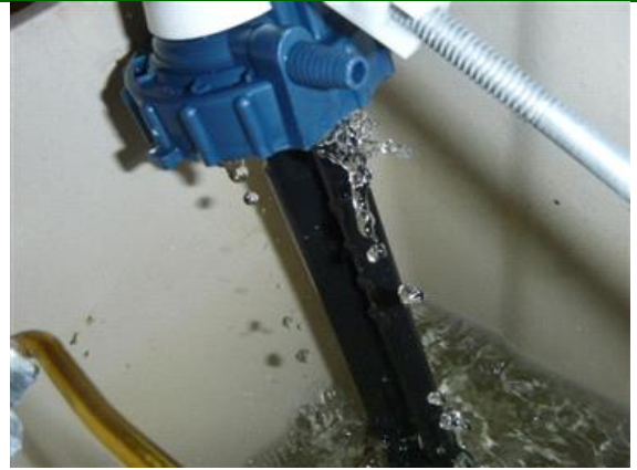
Leak At Bottom Of Toilet Fill Valve
