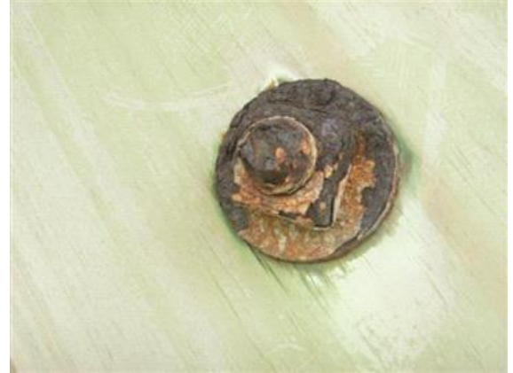
Typical Heavily Corroded Bolt/Nut
