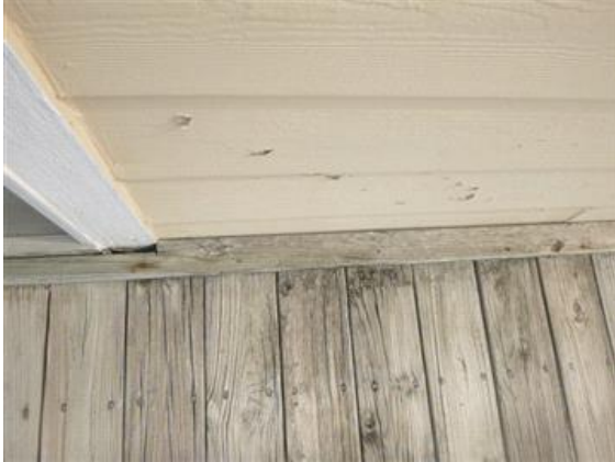
Board Over Deck Connection To The House
