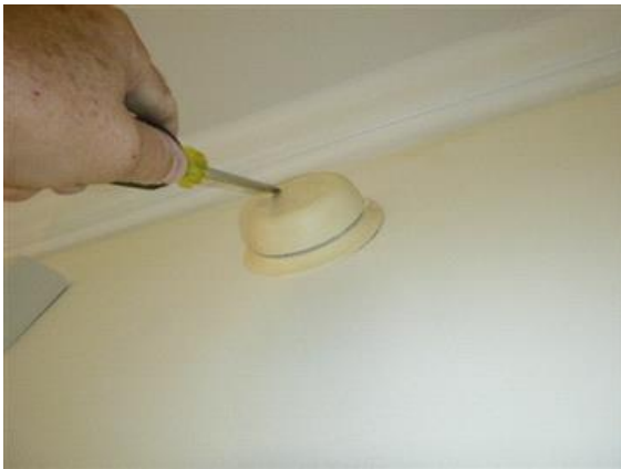
Smoke Detector Test
