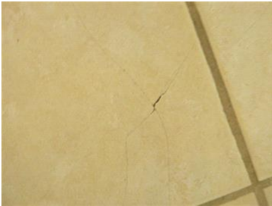
Cracked Floor Tile
