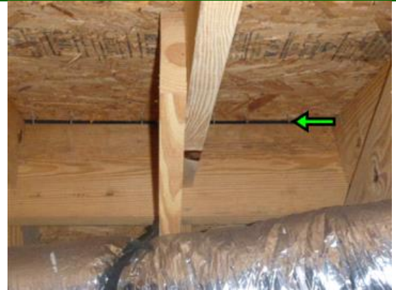
Interior Of Ridge Vent
