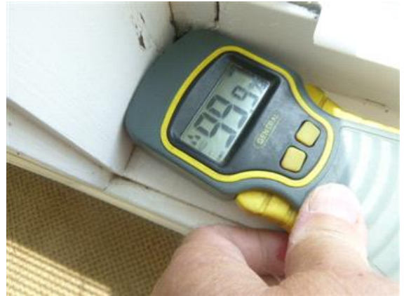
High Moisture Meter Reading
