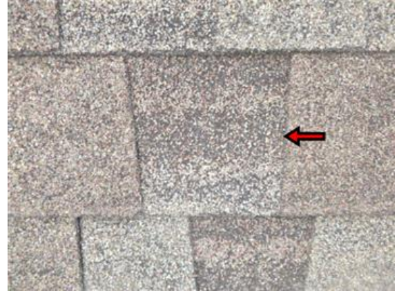
Minor Granular Loss
