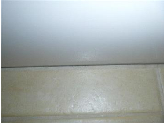
Open Floor Grout Joint at Tub
