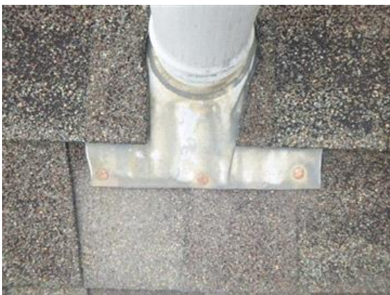
Exposed Nail Heads
