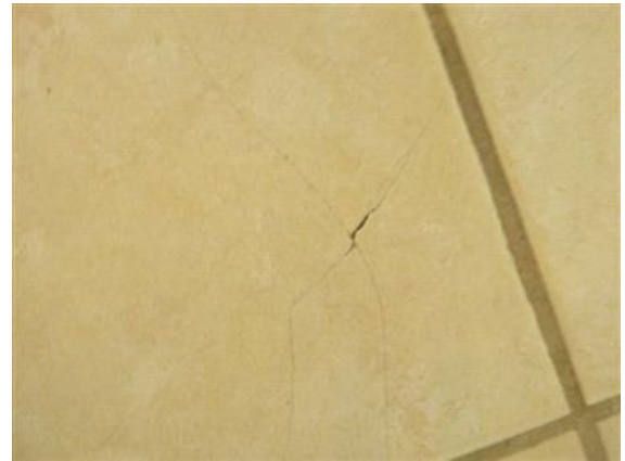
Cracked Floor Tile
