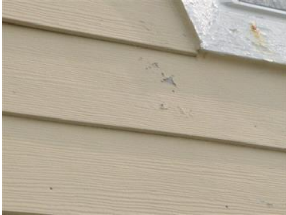
Chipped/Peeled Paint
