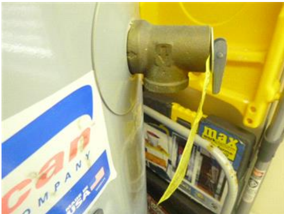
No T/P Relief Valve Extension
