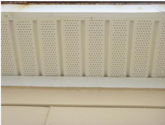
Soffit Vents
