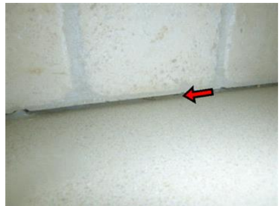
Open Calking/Grout Joint Countertop Back Splash
