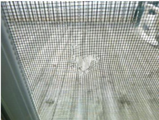
Hole In Window Screen
