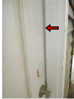
Storage Room Door Not Closing Properly
