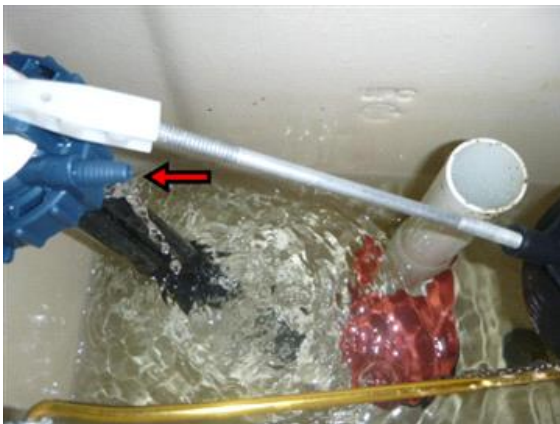
Missing Toilet Fill Tube
